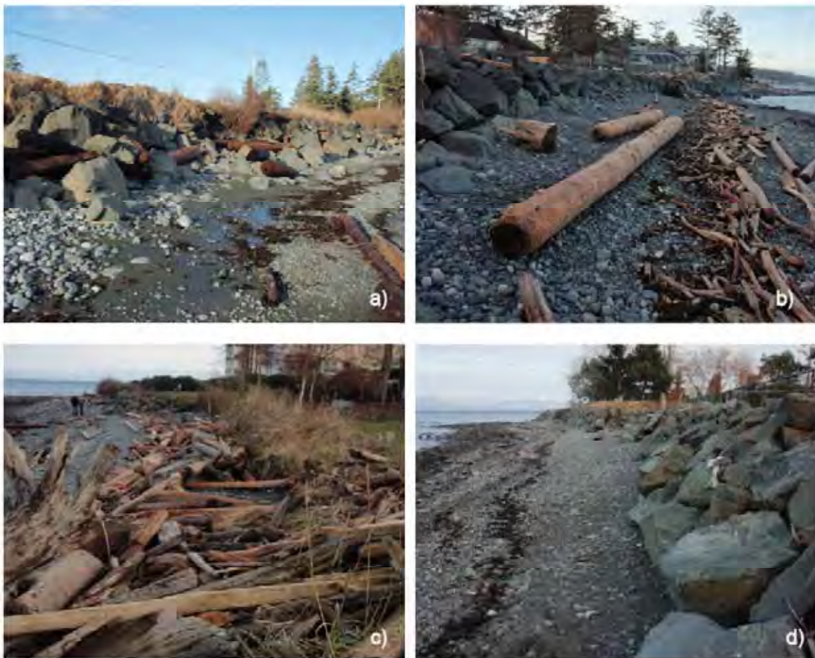
Figure 13. Photos showing conditions at the lower priority sites (see Table 17): a) along shore near Twillingate Road, b) Larwood Park, c) Adams Park, and d) Frank James Park (photos taken 17 January, 2011).
