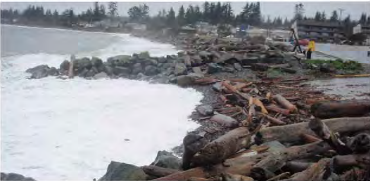
Photo B-2. Sediment and debris depositing on Ken Forde boat ramp during the 31 November 2010 storm.
