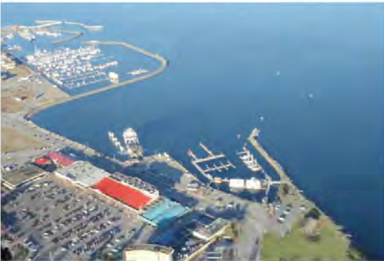
Photo 2. Oblique aerial photo of the breakwaters and jetties installed at the BC Ferries terminal and the Discovery Harbour Marina (photo 18 January 2010).
