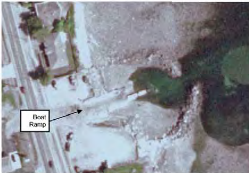
Figure B-2. Aerial view of Big Rock Boat Launch showing rock wings extending from shore (2007 orthophoto).
